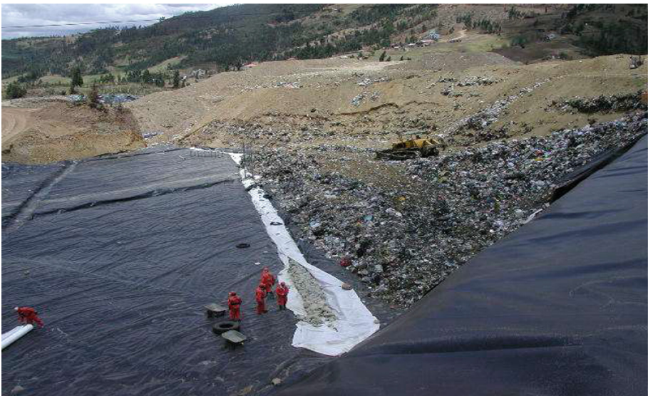
Fig. 20. Conformation and waterproofing of the bottom floor.
