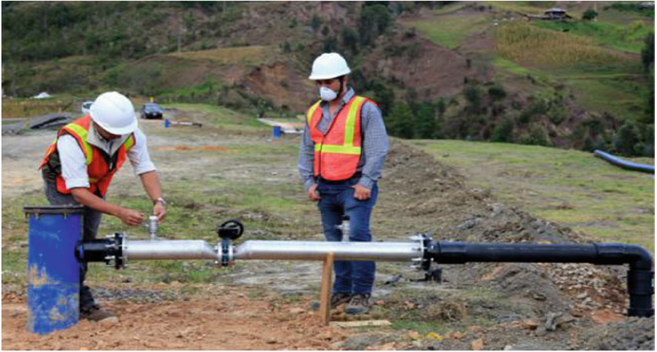
Fig. 4. Regulation of control valves by EMAC EP technicians.
